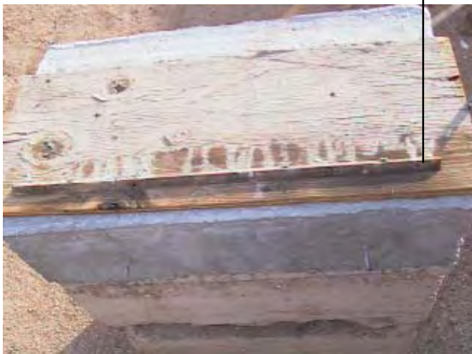
ANGLED METAL BAR ATTACHED TO FORM WORK
