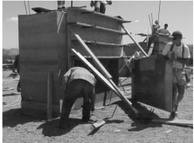
Stripping forms from Gila house.
