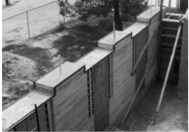
Rammed earth walls under construction for classroom facility.
